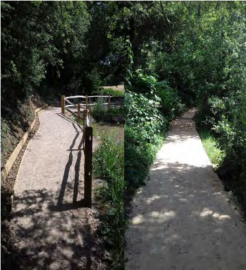
Picture 16 Footpath improvements: surface repair and installation of safety rails near water edge
