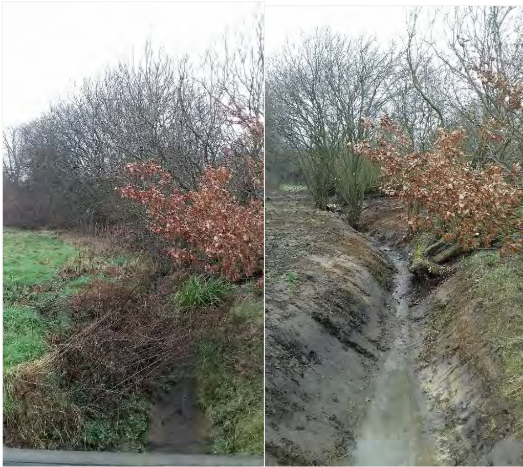
Picture 3 Before (left) and after (right) desilting and scrub clearance along the inlet into lower lake.
