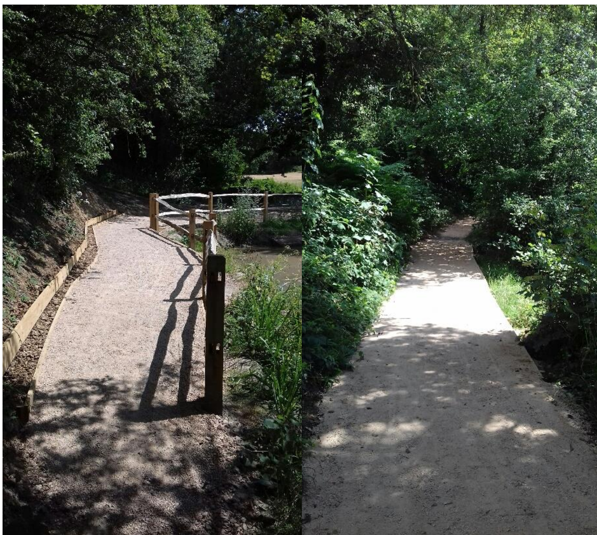
Pictures 19 and 20. Footpath improvements: surface repair and installation of safety rails near water edge
