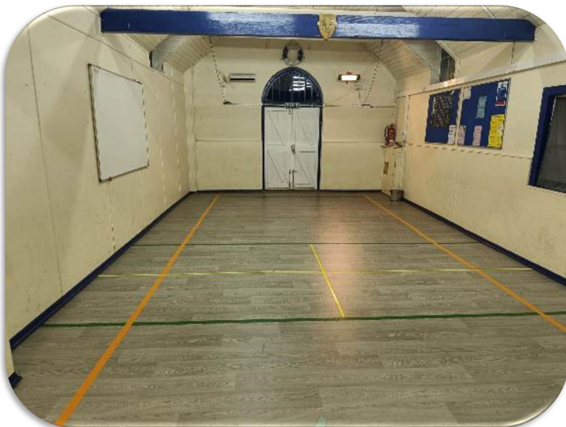
Figure 8: NW121 The repair of the sub-floor, and replacement of the floor surface (Phase 1 of Tadworth Scouts HQ's upgrade) at The Green Hall, Dorking Road, KT20 5SL.
