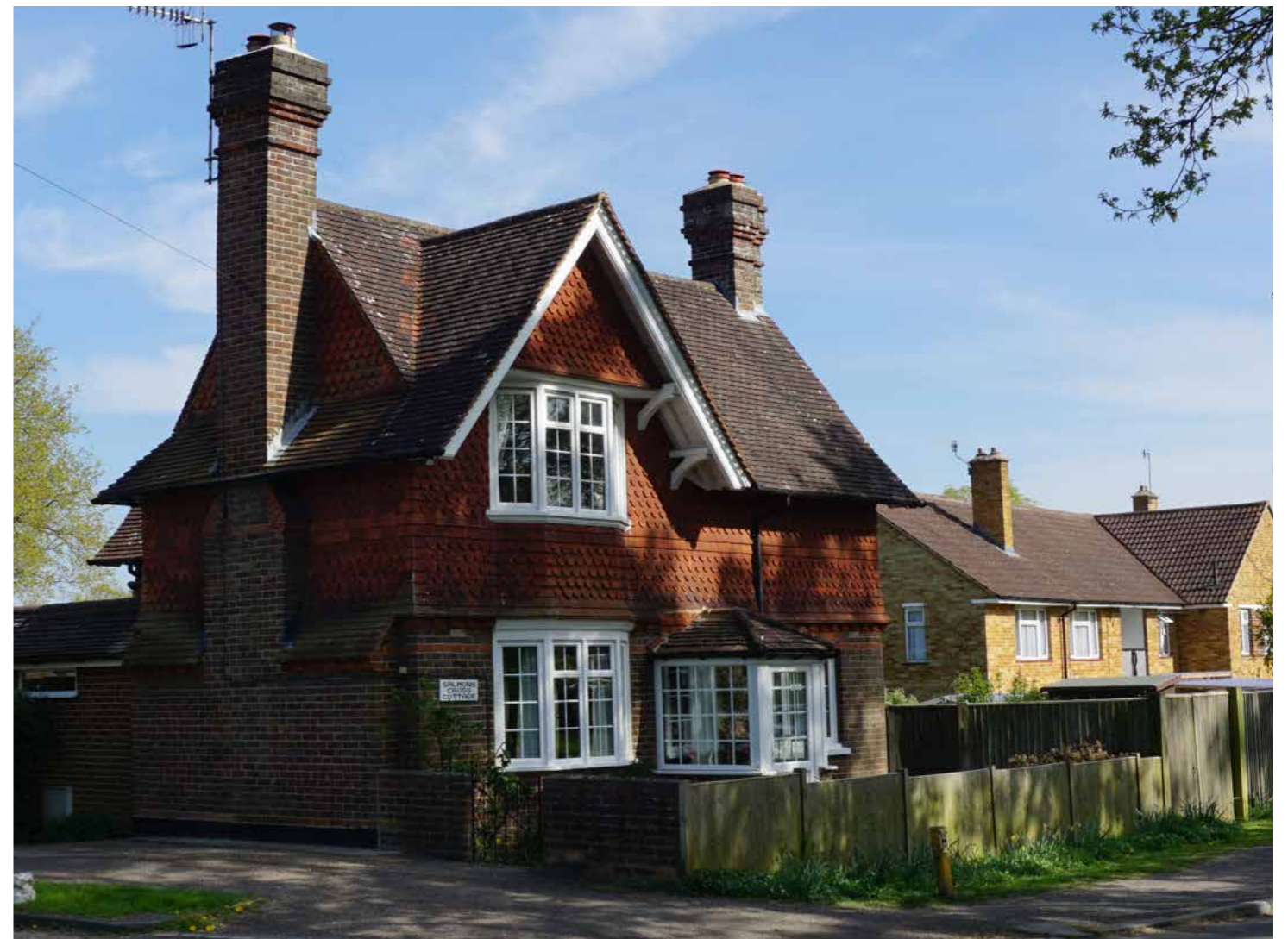
Image 7.3: Stock brick and clay tile hanging
