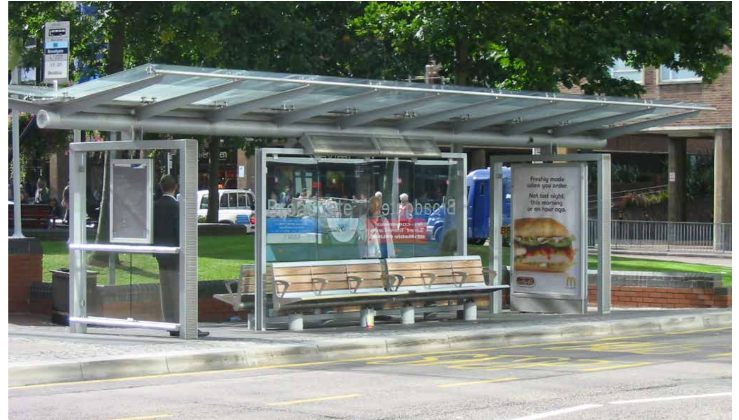
Image 4.6: High quality bus stop shelter
