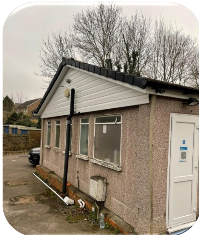
Figure 16: CE62 – New UPVC fascias and soffits, replacement of the guttering at the 7th Reigate Scout Group headquarters building in Redhill.
