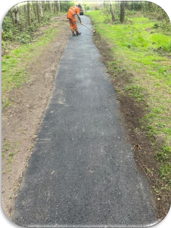
Figure 3: NE32 – Resurfacing of footpath between Hatch Gardens across Burgh Heath
