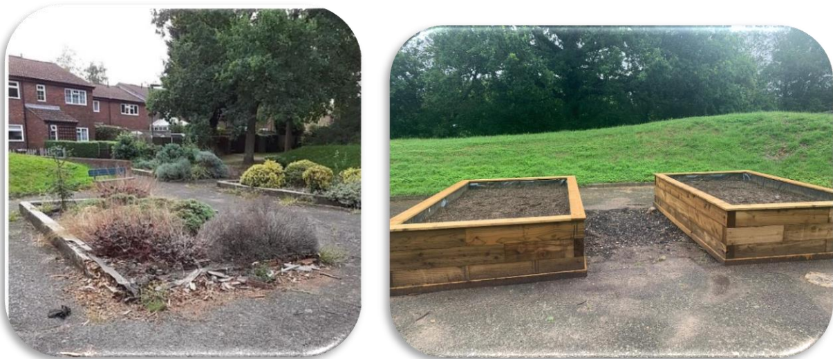
Figure 2: CE51 - Planters at Kiln Walk, Whitebushes (before and after)
