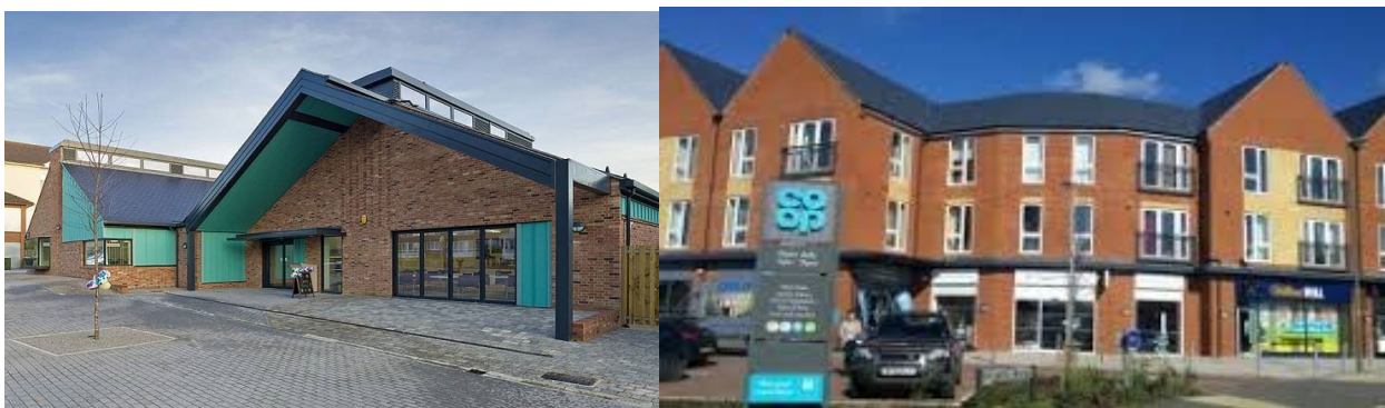
Figure 1 Images of Merstham Community Hub and New Local Centre Shops
