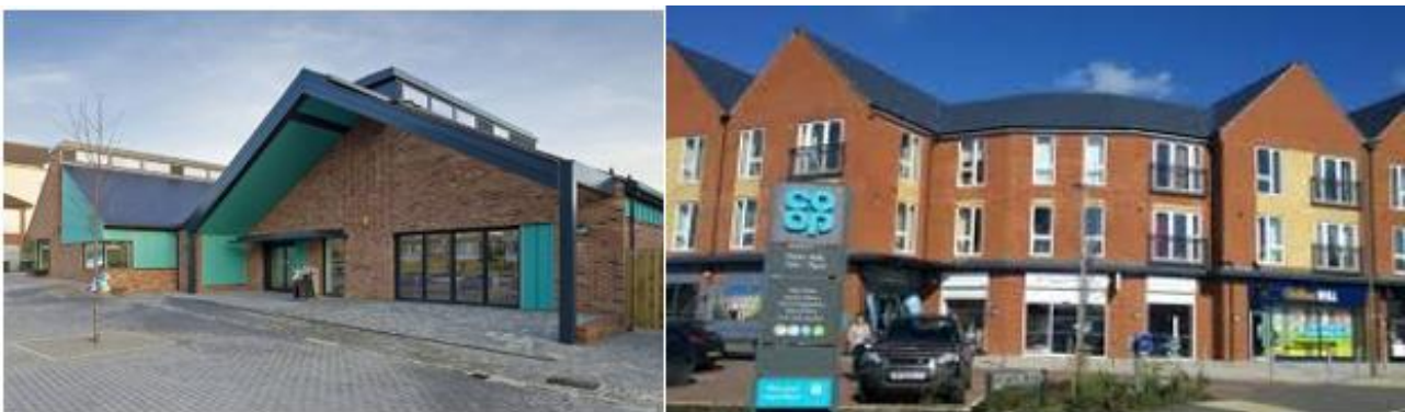
Figure 1 Images of Merstham Community Hub and New Local Centre Shops
