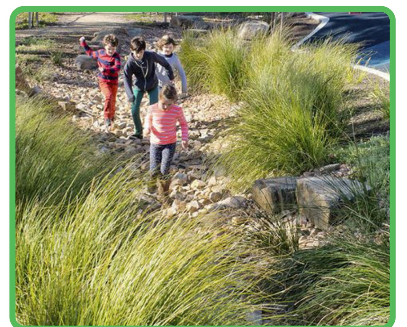
Swales to improve drainage
