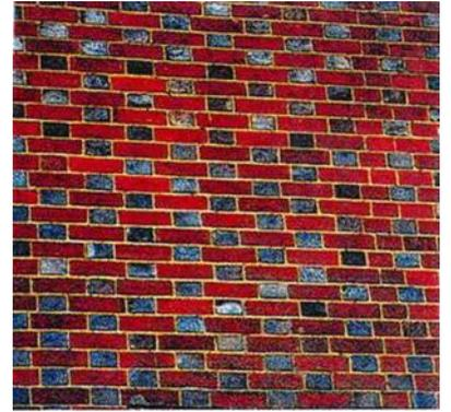
*Figure 71: Flemish bond handmade red brickwork with burnt headers*
