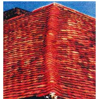
*Figure 73: Handmade sandfaced plain clay tiles with half round ridge and bonnet tiles to hips*
