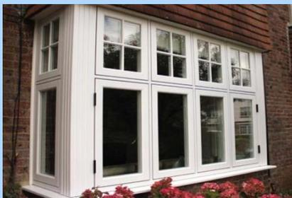
**Figure 87:** A window with equal sightlines would be expected to ensure a good joinery quality to ensure a visually balanced result
