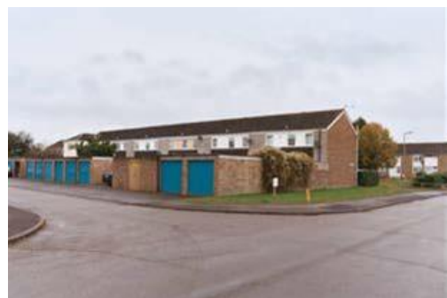
Figure 44: Manor Drive, Horley - a highways dominated layout with separate garage accesses
