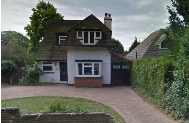
Figure 115: Original house (image source: google maps)
