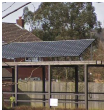
Figure 92: Garden arrays have been used in the borough to reduce visual impact. Image source: Google maps
