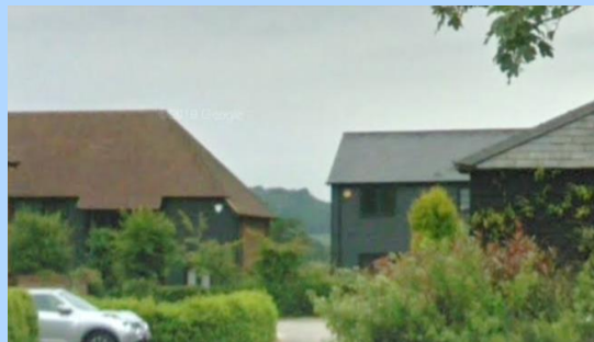
Figure 101: Farmyard conversion at Merstham with historic granary retained to right and new barn like housing to the rear, using traditional agricultural form (no rooflights, no dormers, no chimneystacks, black featheredge boarding and windows minimised).
