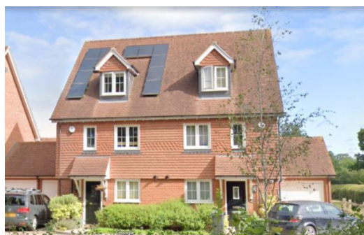
Figure 91: This array has a detrimental appearance due to the asymmetrical stepped appearance and it unbalances the roofscape. Image source: Google maps
