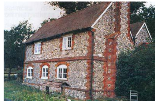
Figure 75: Flint cottage; flint is generally found north of M25
