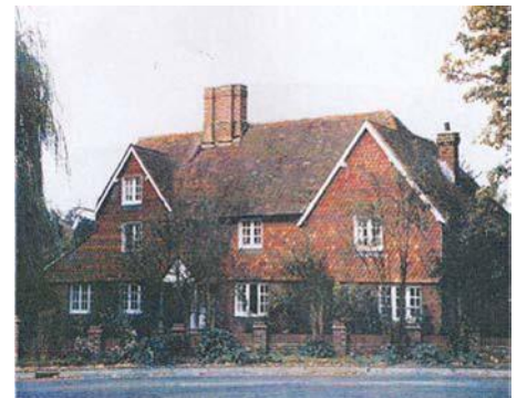
Figure 80: Typical asymmetrical Wealden vernacular farmhouse 50 degree pitch clay tiles and decorative tile hanging
