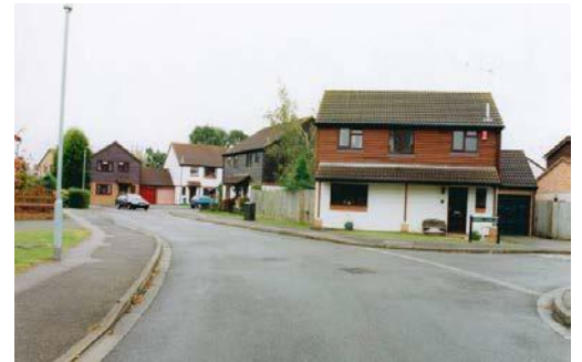
Figure 76: Parkhurst Road, Horley - painted timber boarding does not reflect materials used historically
