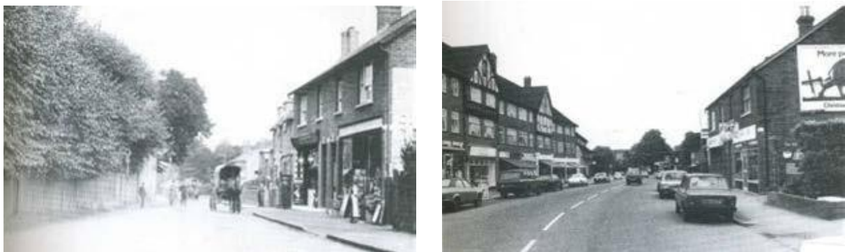
Figure 14: Banstead High Street 1910 and circa 1987 illustrating Loss of Village Character Source: Banstead Then and Now Photographs courtesy of Banstead History Research Group
