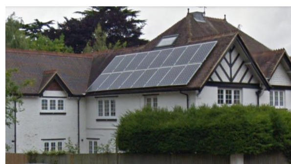
Figure 90: This panel is obtrusively placed on the south east front of a house when the south west rear place would have been a possible location. The silver frames and lack of integration into the roof add to the prominence of the panels. Image source: Google maps.
