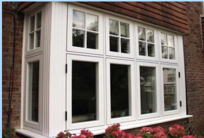
Figure 86: A window with equal sightlines would be expected to ensure a good joinery quality to ensure a visually balanced result
