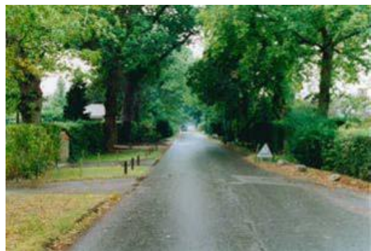
Figure 34: Haroldtslea Estates, Horley - buildings set back behind mature avenues, carriageway has no kerbs
