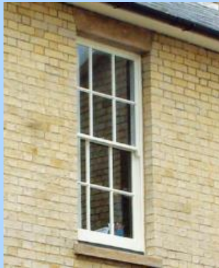
Figure 89: Sash windows should be vertically sliding. The proportion of the window opening and panes should have a vertical emphasis with the window opening following the double cube proportion. Sash should generally be set back behind the reveal (unless exposed box sashes).
