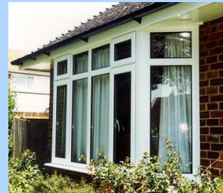
Figure 85: Unequal sightlines are harmful to the appearance of a building as they lack harmony and balance.
