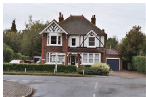
Figure 29: Massetts Road, Horley - Conversion of villas to other uses results in loss of large front gardens to hard standing for parking
