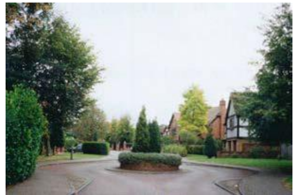
Figure 47: Harendon/ Mabbots, Tadworth - road layout includes over-engineered traffic calming measures
