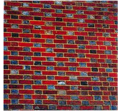
Figure 69: Flemish bond handmade red brickwork with burnt headers
