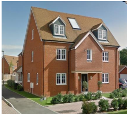
Figure 94: Centrally placed panel. Image source: Google maps.
