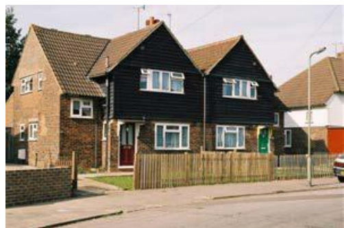
Figure 40: Brook Road Merstham - example of weatherboarding, painted a dark colour
