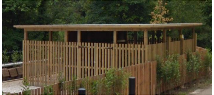
Figure 96: The location and cycle and bin stores should be considered before submitting plans and carefully screened by planting. In this particular case, the forward location and tall roof structure has made this design more detrimental.
