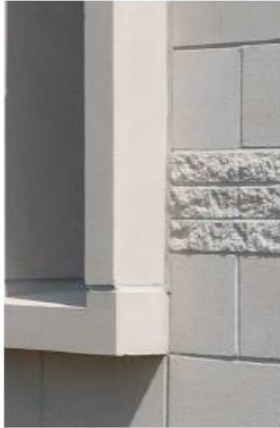
Ivory fair-face smooth concrete block with courses of split-face ivory linear blocks
