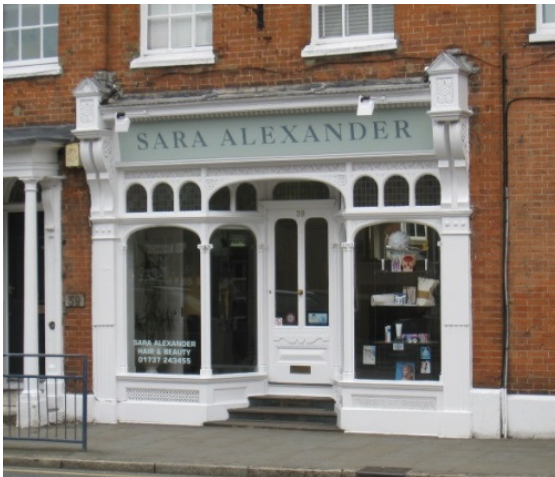
A restored Victorian shopfront in Reigate
