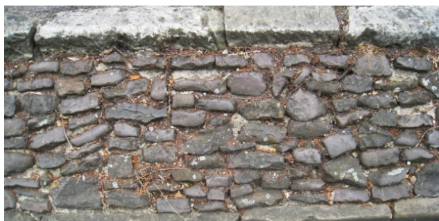
An 18 th century ironstone pavement comprising large Purbeck stone setts and thin Yorkstone kerbs, restored as part of the Home Zone Scheme, Reigate
