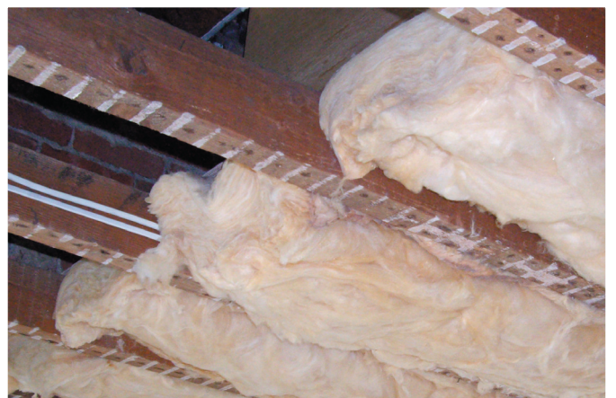
Loft insulation being installed
