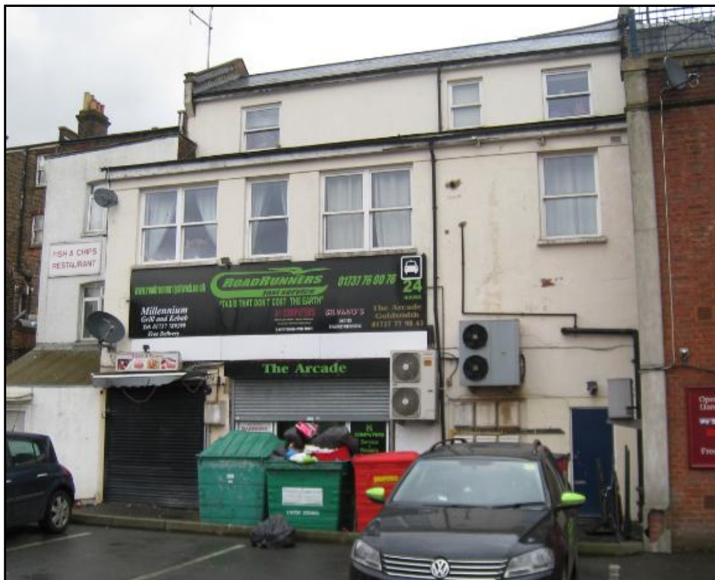
Figure 16: Rear of Station Road
