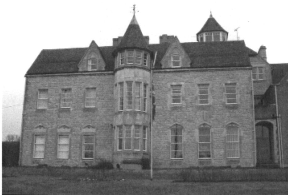
St Davids, a house by 1860, was founded as a school in 1882 which survived till 1939. After the war it became a part of the Surrey Fire & Rescue Headquarters.
