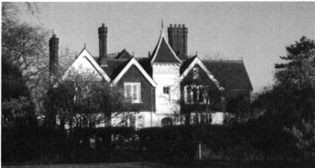
Wraylands is a substantial Victorian house of the 1850's with tile hanging typical of the area and a prominent turret.
