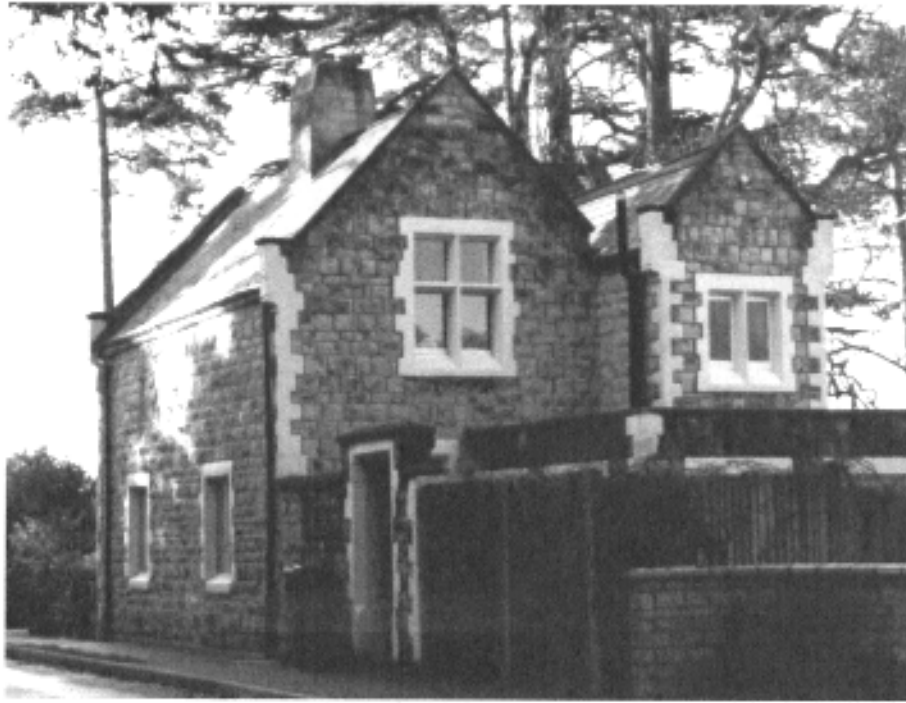
Further on is Little Gatton Lodge , built in Reigate Stone in the 1850's.
