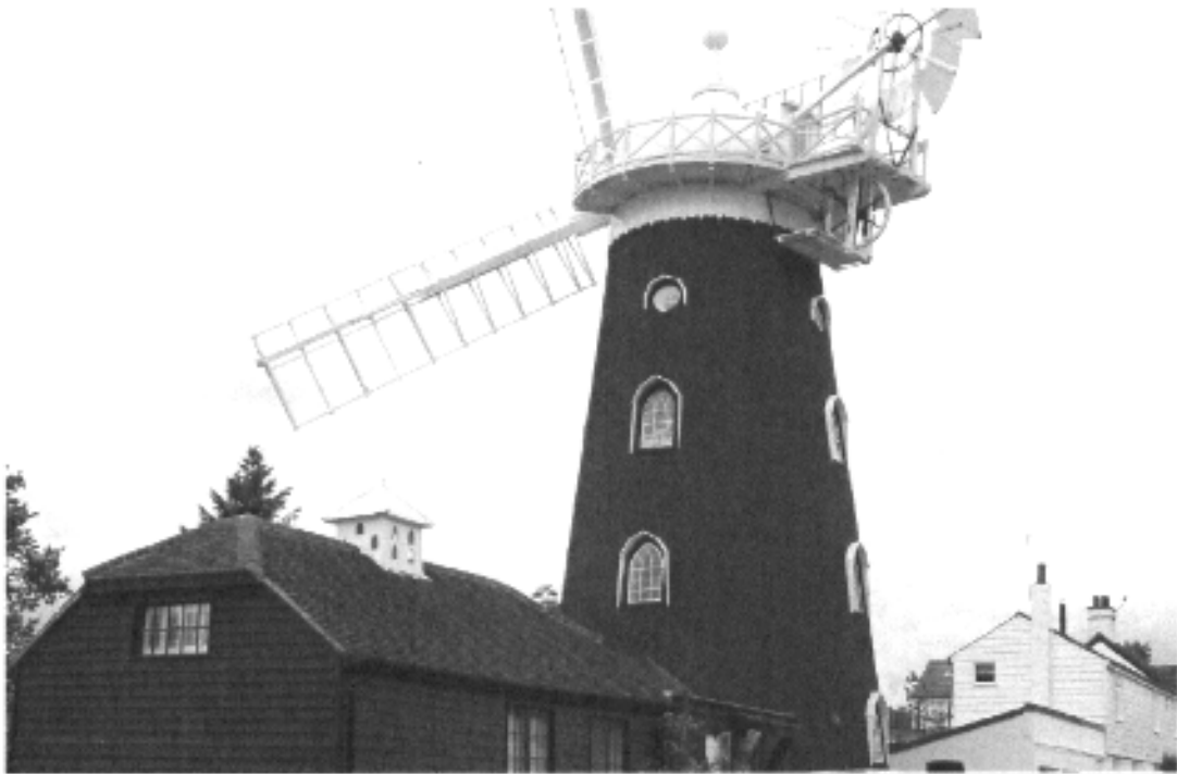
To the north west is the black tarred tower Windmill of 1824, a local landmark, with its granary on staddles and weatherbaored Miller's Cottage.
