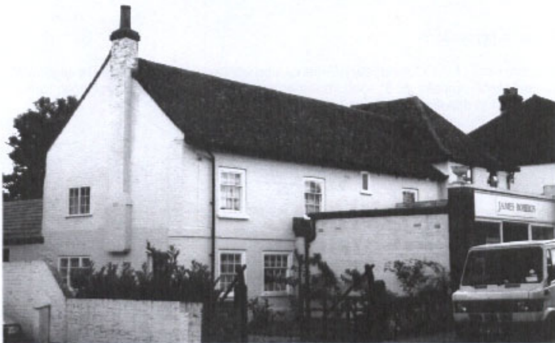
Statutory Listed Building in Walton Street which could benefit from removal of bungalow shopfront
