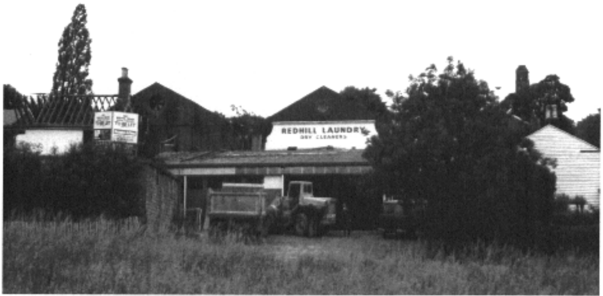
The Redhill Laundry site, now Ardshiel Drive.
