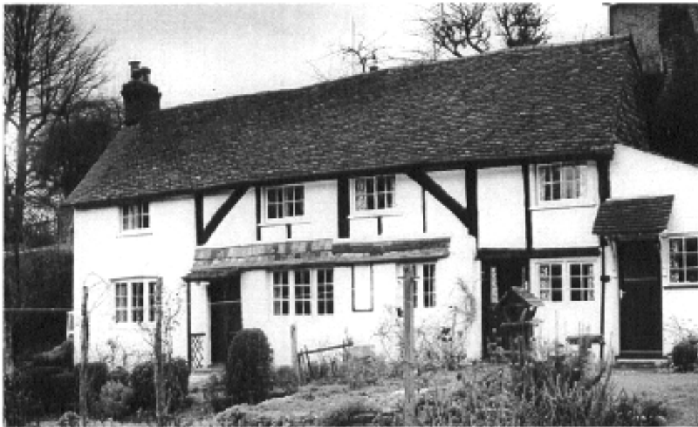
10 & 11 Pendleton Road, an early 17 th century timber framed house (SHC)
