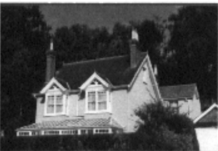
4 pendleton road, a house with early origins but extensively rebuilt in the late 19th century
