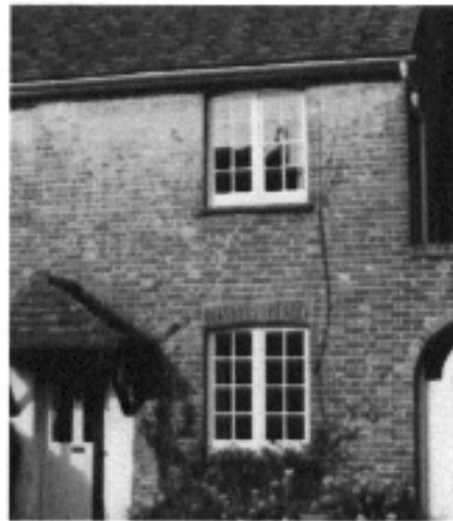
Flemish Bond brick with burnt headers
