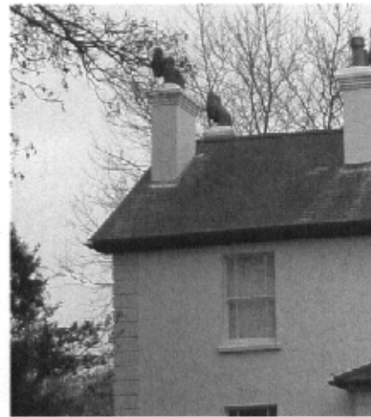
Stucco with slate
