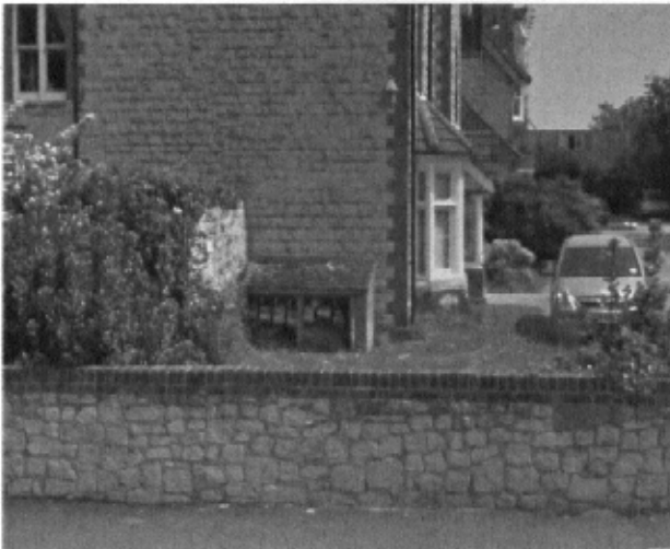
A Reigate Stone wall
