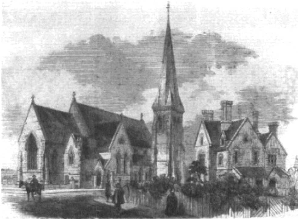
St Marks Church 1861
