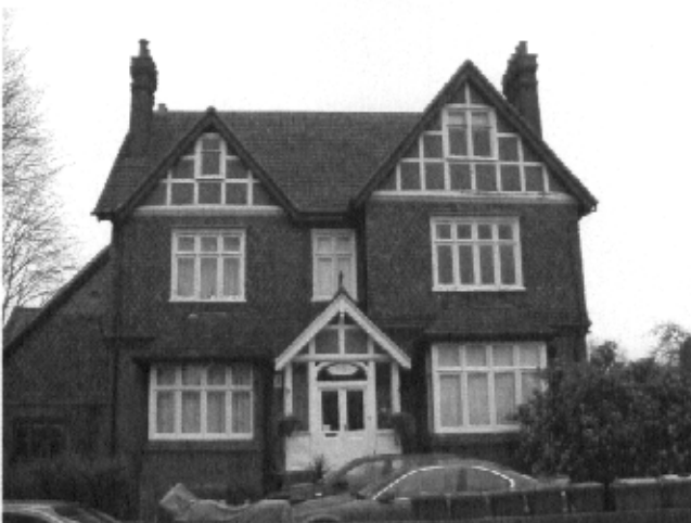
Late Victorian Tile Hung Old English style properties with handmade clay plain tile roofs and mullin and transom windows
