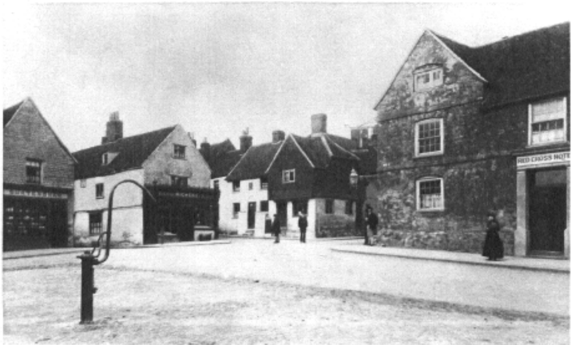
The west end of the High Street in the 19 th century. Slipshoe house is behind the cottages later demolished for road widening. The Red Cross is seen with its Georgian sashes and brickwork, before the Edwardian windows and roughcast were added.
