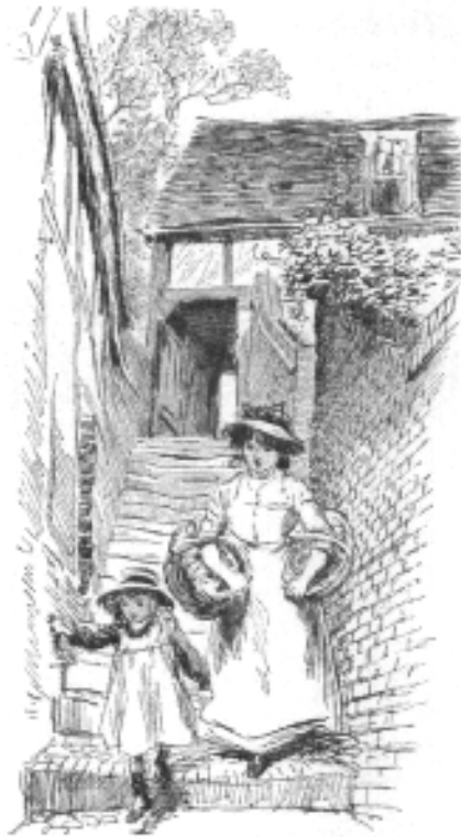
The Crown Steps or Donkey Steps, High Street, Reigate. A landmark of the town, the ironstone steps are set wide for the horses which accessed the stables, now cottages at the top of the steps. The County have programmed repairs for the steps in 2016.
