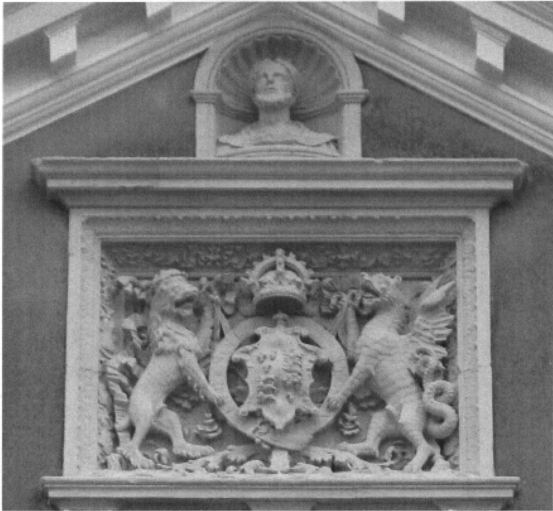
A bust of William Howard, 1st Baron Howard of Effingham (c. 1510 – 12 January 1573) the first residential owner of the Priory with Henry VIII's coat of arms in the pediment of the Priory. These carvings were probably originally situated in the gatehouse of the Priory which would have been located in the vicinity of the sunken garden.
