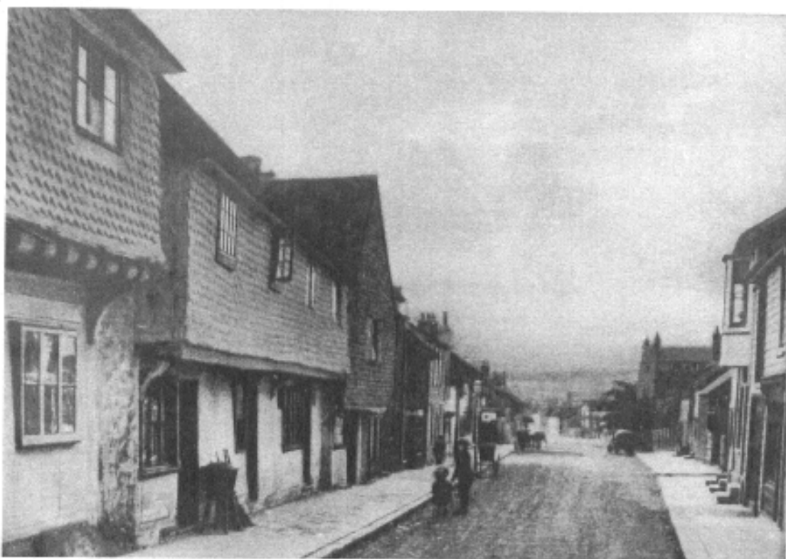
West Street in the late 19 th century with the tile hung cottages which are a distinctive feature of the town.
