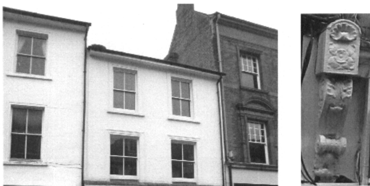
The painted stucco buildings in Station Road West are the oldest surviving shops within the area, built around 1859. They are characterised by a classical proportion and the use of sash windows set back behind the reveal. The shopfronts were originally defined in terms of their fascia height by console or corbel brackets.
