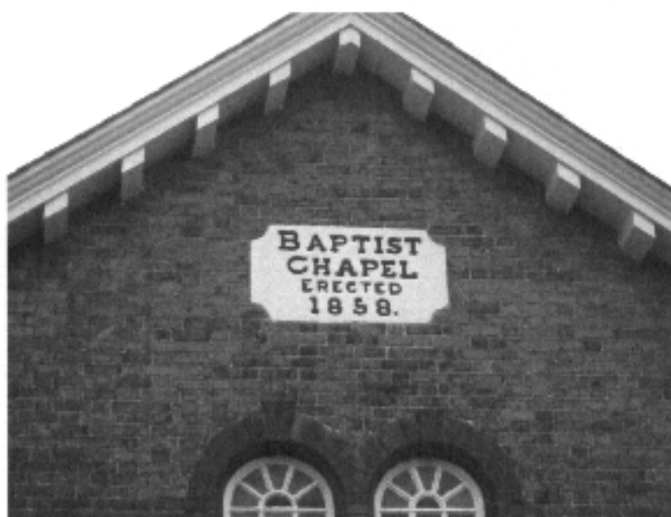
The Baptist Chapel in Station Road West has London Clay stock brick with red brick dressings. Pevsners Buildings of England notes the traditional lettering. The windows are cast iron.
