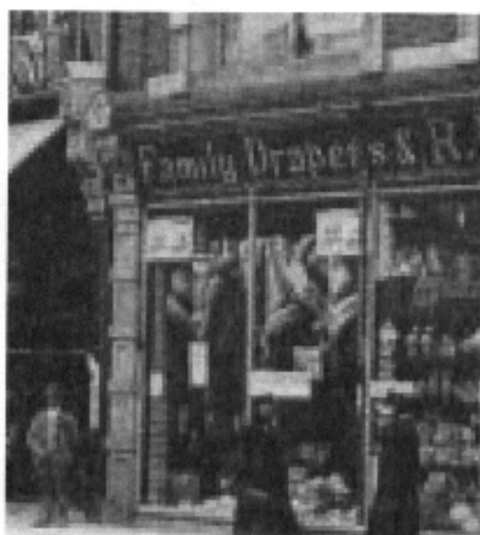
Oversized fascia at 34 Station Road with the capitals indicting the correct proportion for the fascia
