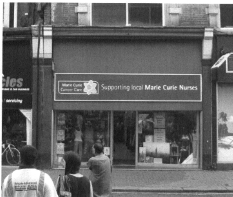
Oversized fascia at 34 Station Road with the capitals indicting the correct proportion for the fascia
