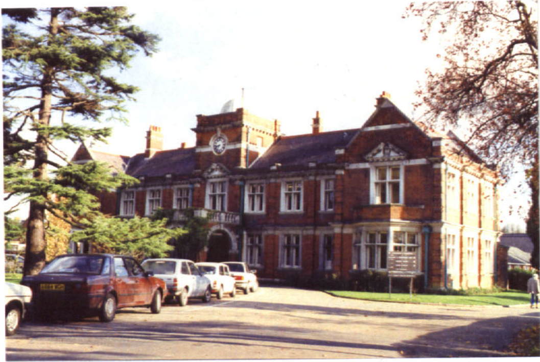
The Administration Block
