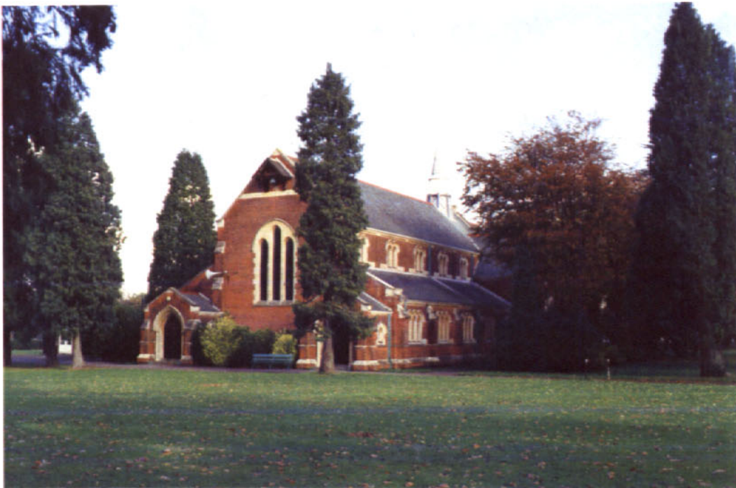
The former Chapel
