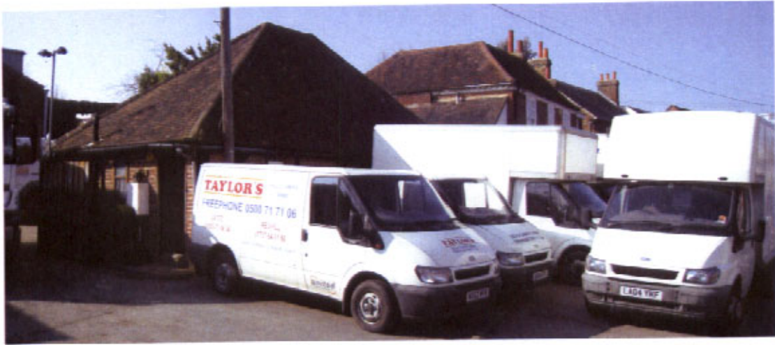
On the east side the remains of the former thatched barn are lost within the collection of vans
