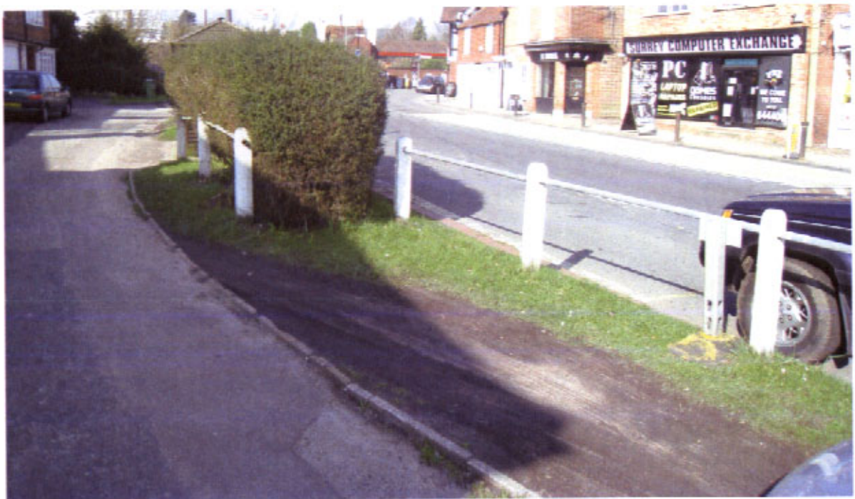
Erosion of the grass verge due to parking
