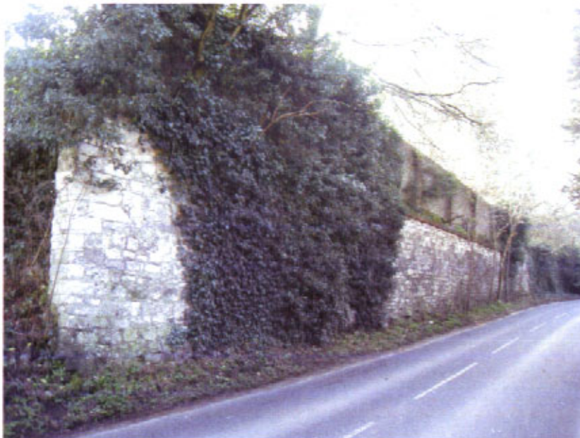
This stone wall was built to provide a flat lawn to Merstham House and a base for a kitchen garden wall above
