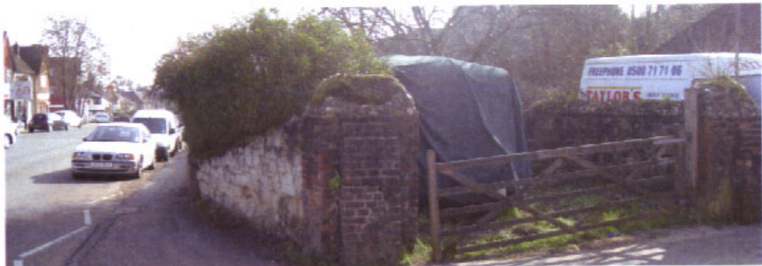
The poor condition of the village pond has been raised with the Hylton estate.
