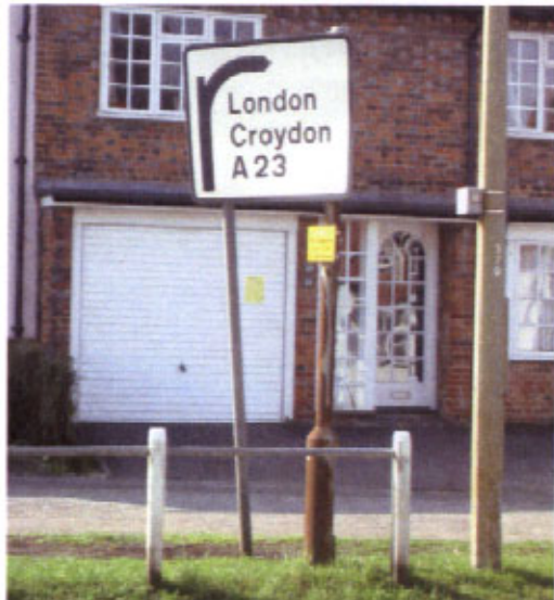
A distorted and rusting street sign detracts from the character of the grass verge.
