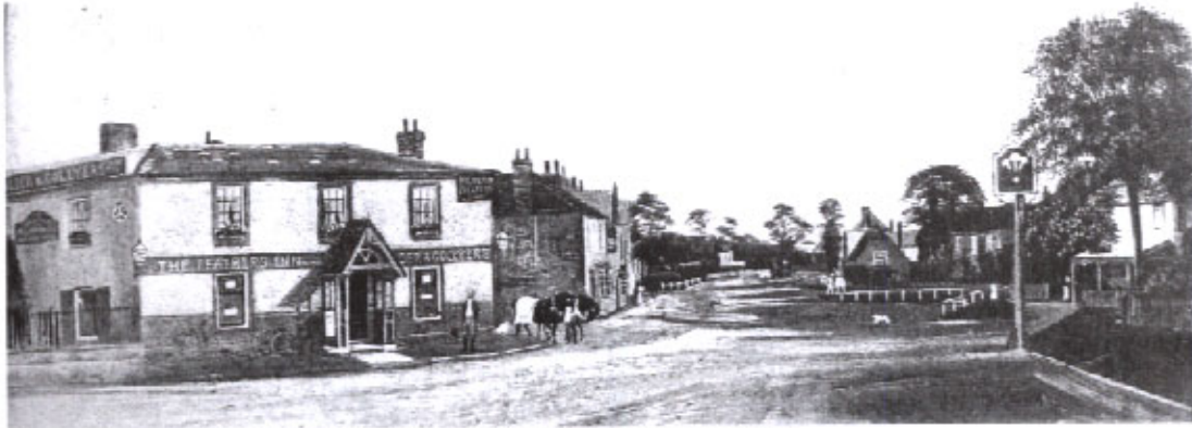
The village before the rebuilding of the Feathers in 1895
