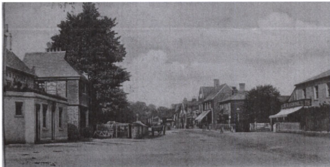
The Cottage of Content public house, now a dwellinghouse, the village pound and blacksmith and the old thatched barn c1903
