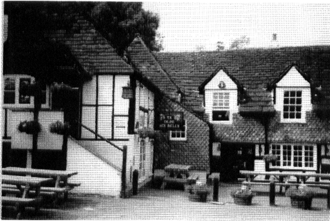
The 6 Bells illustrates the materials found in the area such as Horsham Slab, decorative tile hanging, timber frame, painted brick as well as sash windows and casements.
