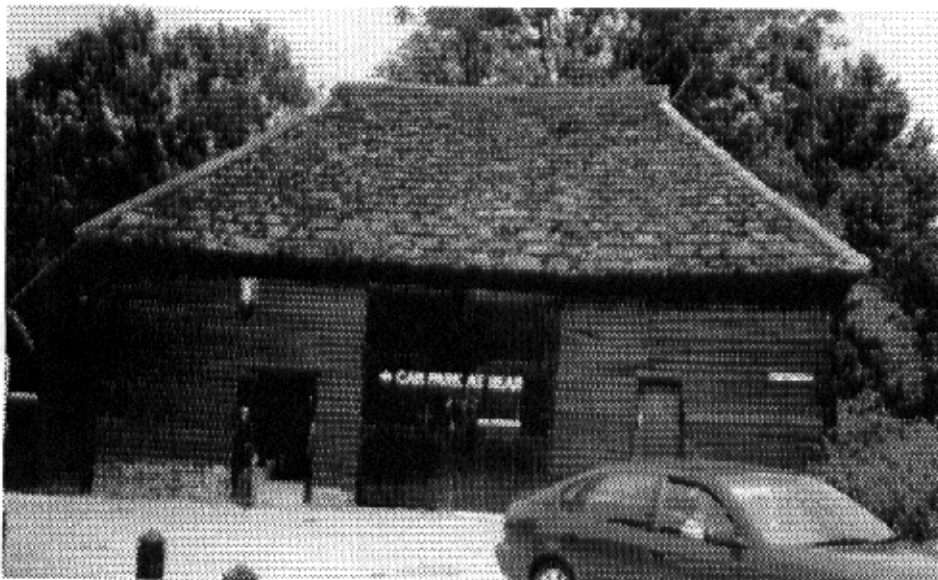
The Barn to the 6 Bells shows the the use of black stained feathered edge weatherboard and has someperiwinkle stone to the plinth.
