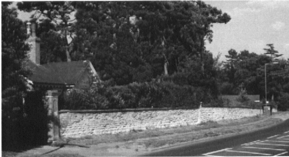
The Victorian Reigate Stone wall to Buckland Road is a distinct and prominent feature.
