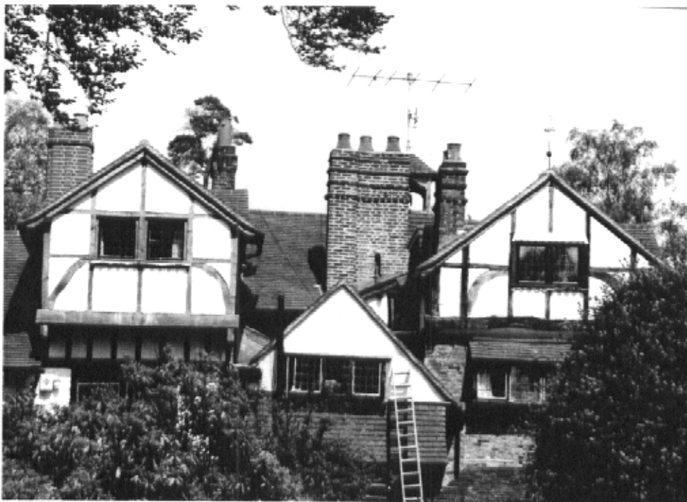
The Cottage, a good example of Garle picturesque architecture
