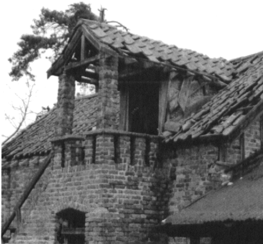
Outbuilding at Russian Cottage before conversion to a house
