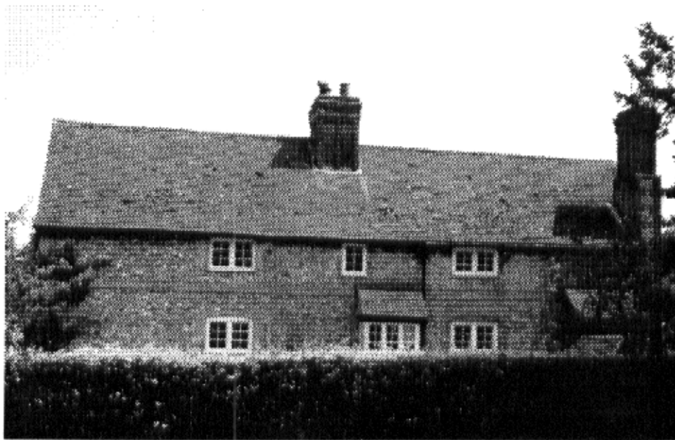
Ruffetts Cottage, a 17th century flint cottage of early central chimney form
