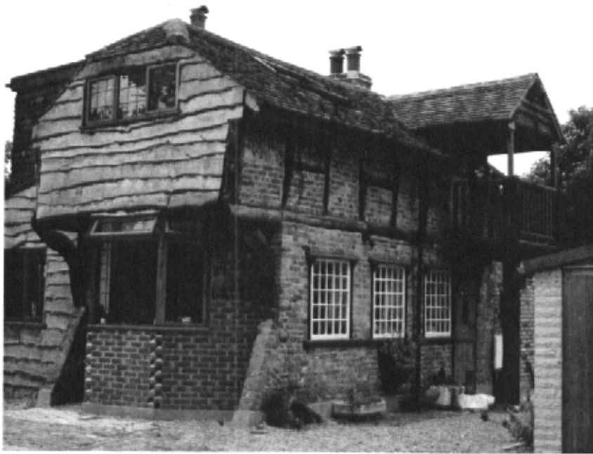
The Keep with bad later infill at ground floor
