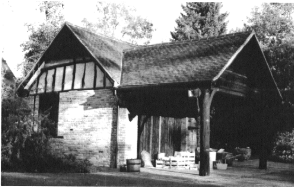
Ruffetts Wood in 1989 with outbuilding below, a good example of Garle use of irregular timber frame and pine pole timbers for supports.
