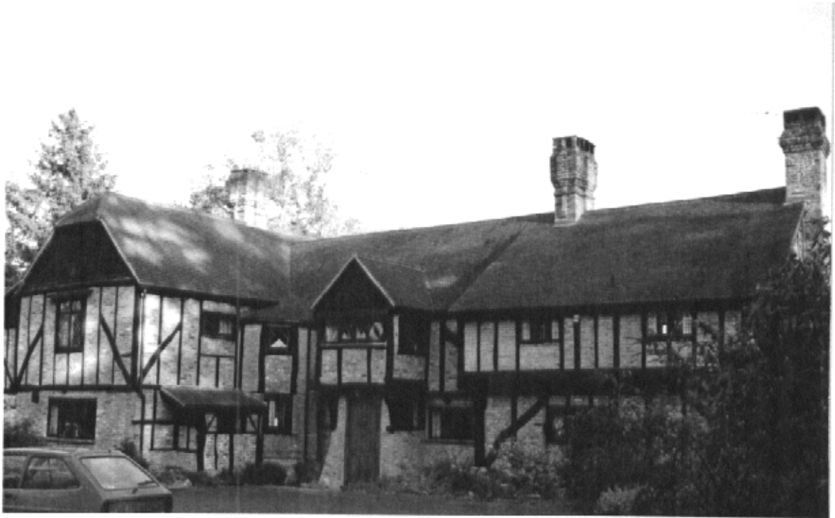
Ruffetts Wood in 1989 with outbuilding below, a good example of Garle use of irregular timber frame and pine pole timbers for supports.
