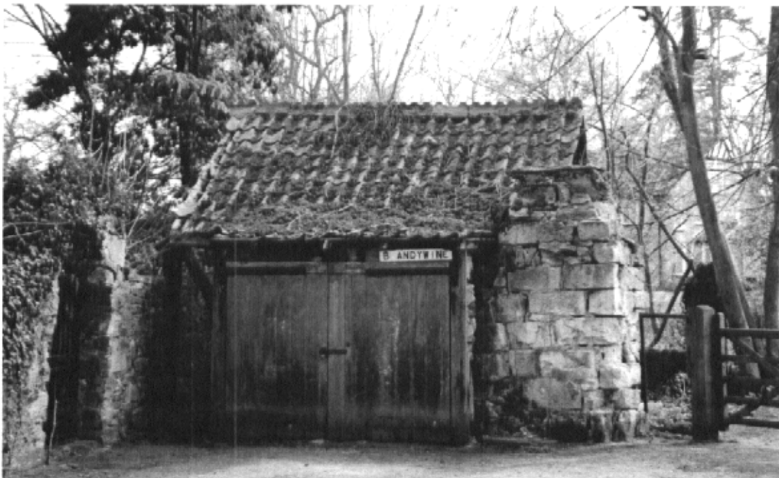
Garage at brandywine before partial rebuilding, showing the chalk blocks, which lost some of their character in rebuilding.
