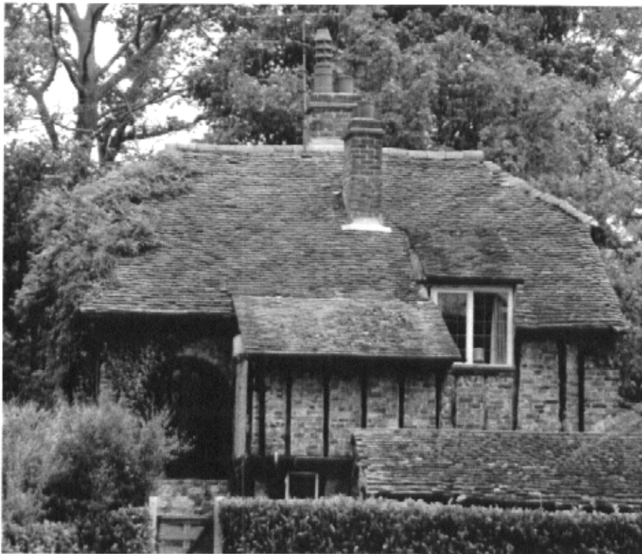
Farm Cottage, a good example of the Garle irregular use of materials and bonding
