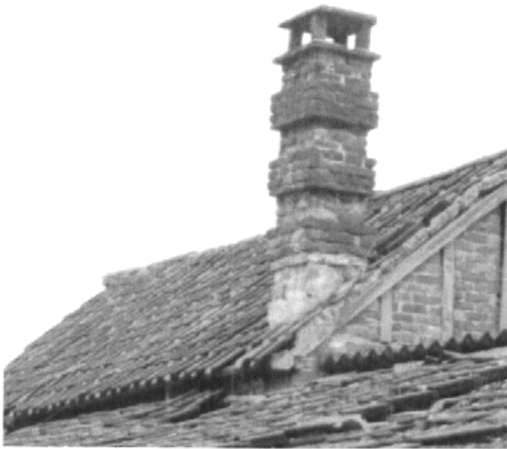
Example of a Garle chimney, at an outbuilding at Russian Cottage.
