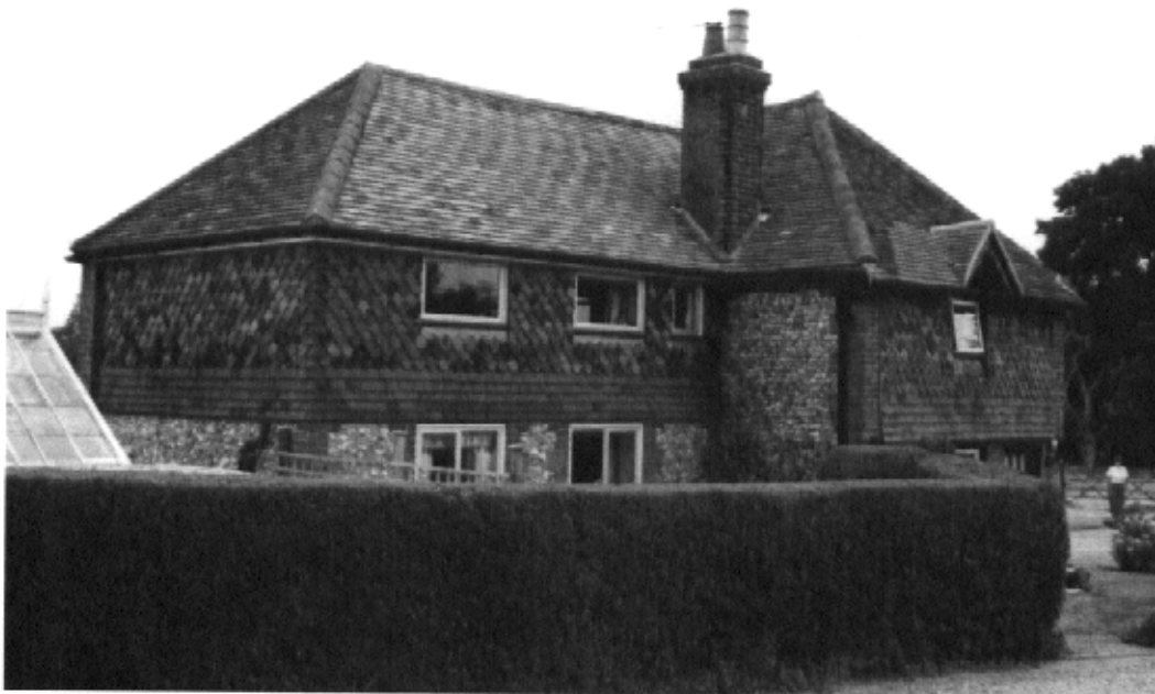
Court Lodge Cottage 18 th century flint cottage with Victorian additions in the 1980's. The inappropriate aluminium windows have been subsequently replaced.
