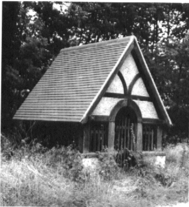
Wellhouse, High Road of the 1870's by E.M. Barry
