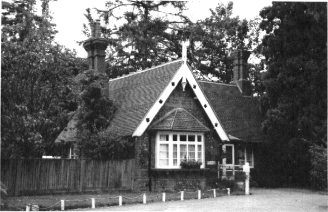
Elmore Lodge, a mid 19 th century flint building, the main house behind rebuilt in the 1930's.
