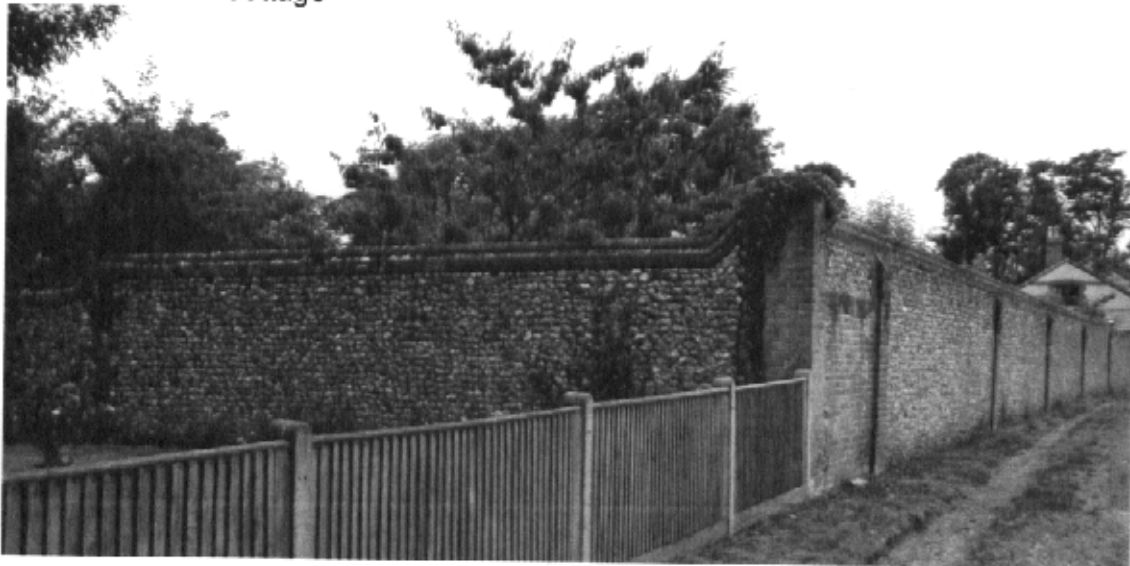
Kitchen garden wall
