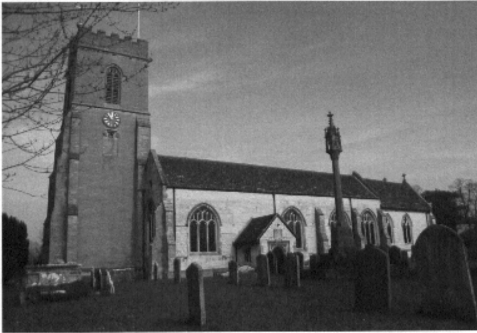
South view of the church with Victorian Churchyard Lantern Cross in foreground, a memorial to the Freshfield family. The Reigate Stone church has suffered from inappropriate refacing in machine cut bath and Portland stone which damage the rural and local character of the church. Aside from this, Reigate is one of the five largest medieval churches in Surrey and is an imposing structure. It is the most substantial surviving medieval building in the Borough and one of the Borough's most important historic buildings.
