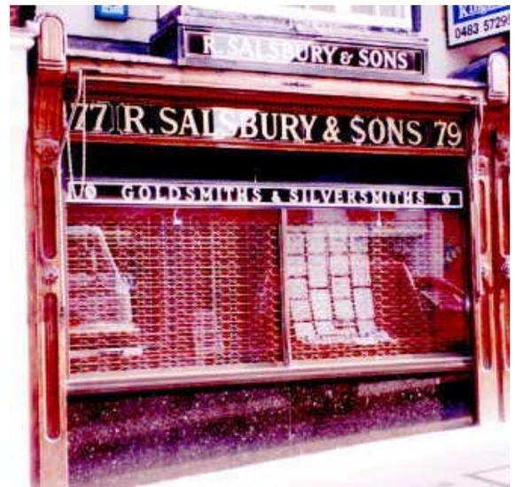
*An internal mesh grille can be both effective and avoid the creating the desolate environment of solid shutters at night.*
