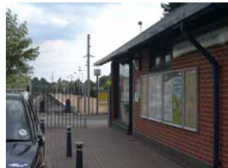
Tattenham Corner Station, Preston's nearest railway station
