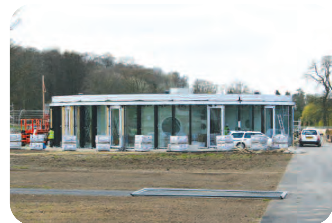
Building in progress
