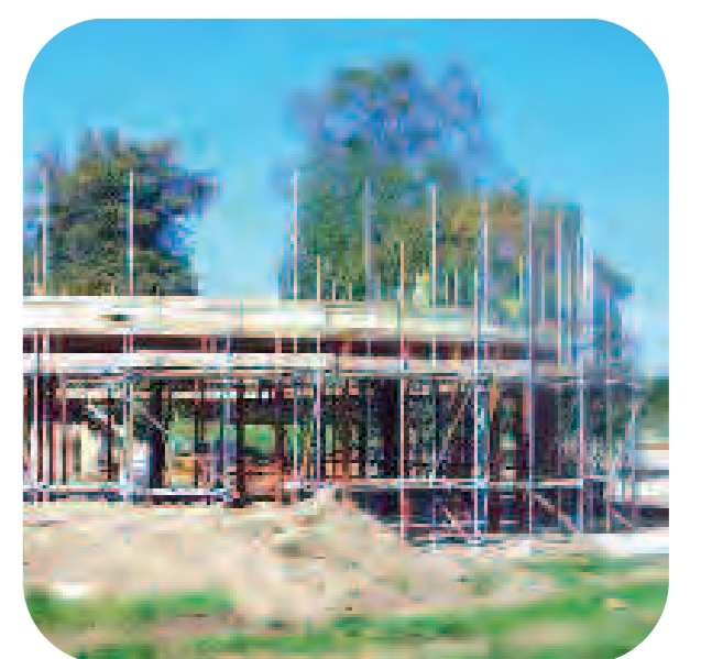
Construction of The Pavilion
