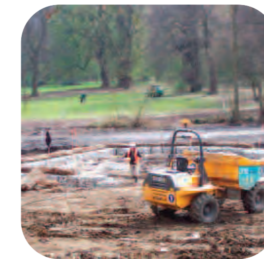
Dredging the Lake
