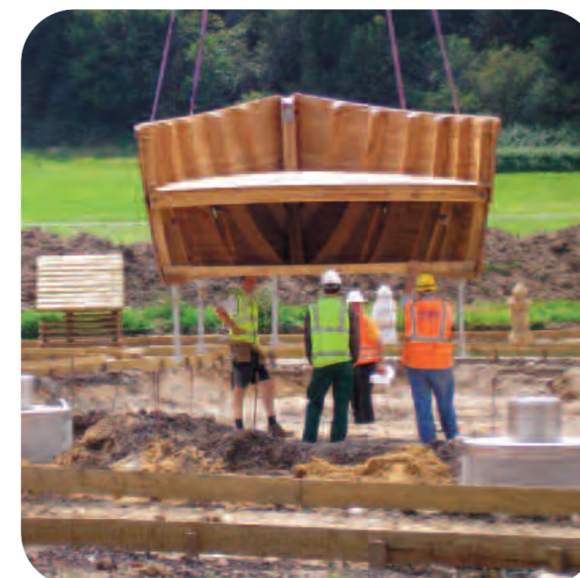
Play area installation
