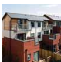
Family Houses, Didsbury Point, Manchester 2004
