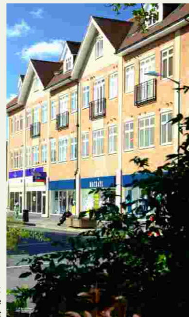
Photo: McKay's store in Horley High Street
